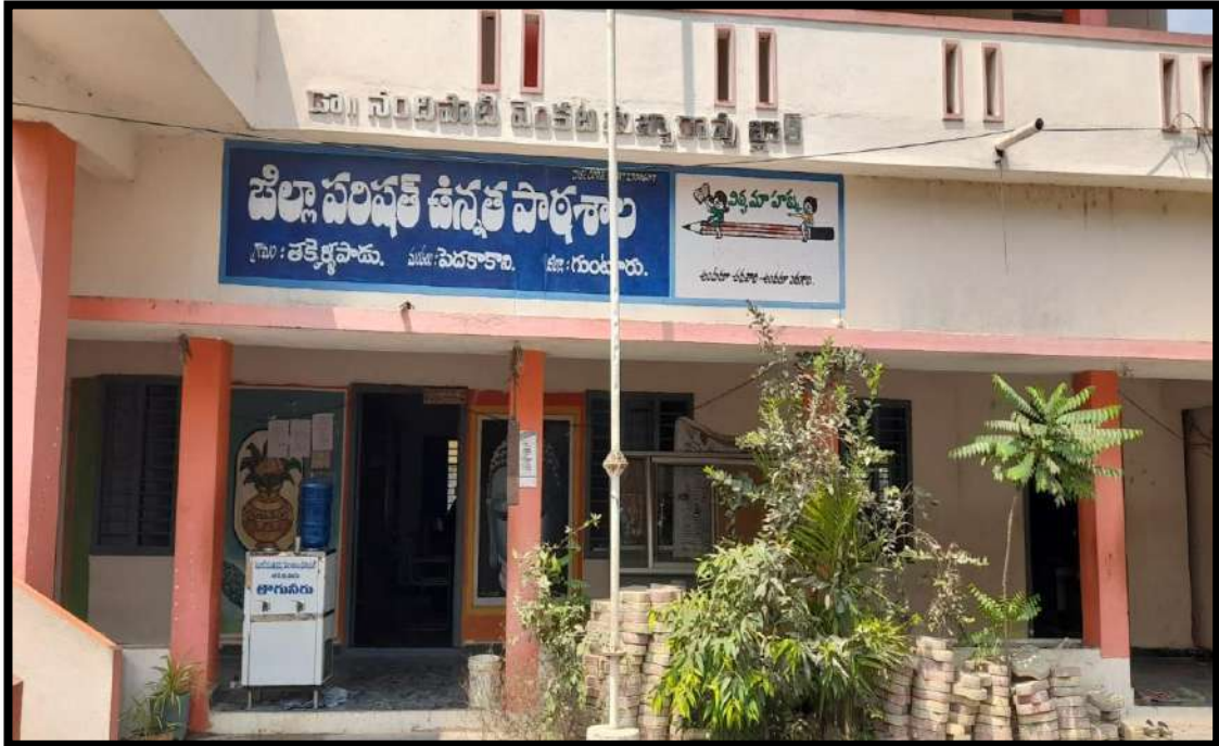
INSTALLATION OF WATER COOLER IN ZILLA PARISHAD HIGH SCHOOL, TAKKELLAPADU
